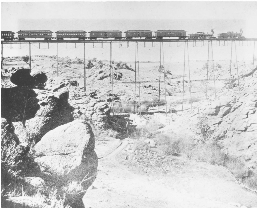
Steel Dale Creek Bridge
