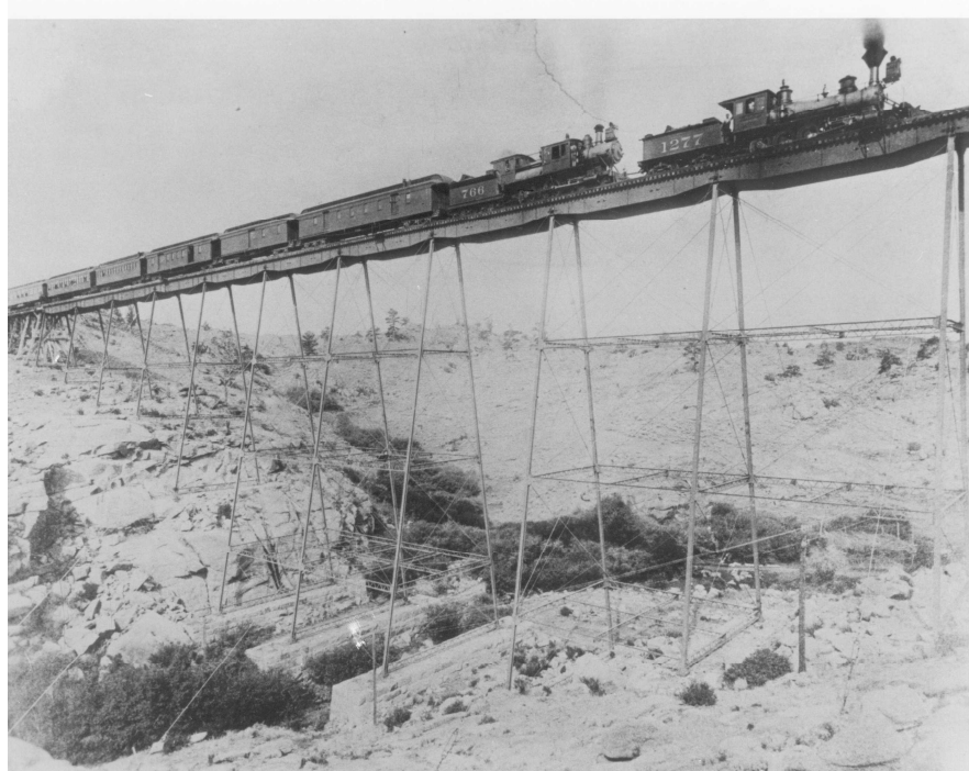
Dale Creek Bridge constructed with steel girders
