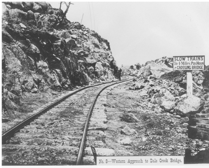
Western approach to the Dale Creek Bridge
