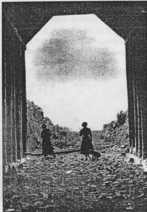
The light at the end. Shown is the Butte Royal tunnel in 1914, shortly after completion. It measured 18 feet in height and 350 feet in length.
